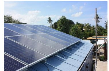
**Taiwan funded solar panels installed on the roof tops of the government office building has a capacity to generate 30360 watts of solar power**
