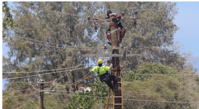
Linesmen hard at work to maintain safe and efficient power supply
