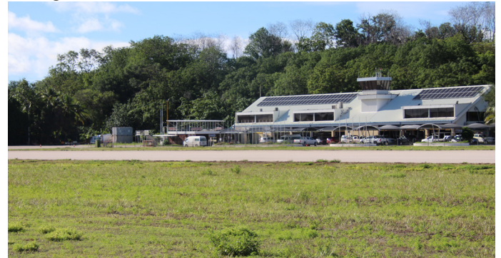
Project to detect UXO is underway for runway upgrade
