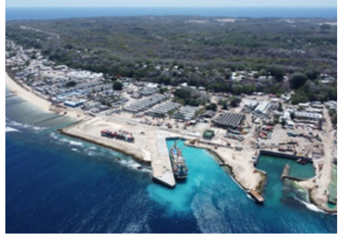
Port commenced operations in 2022, but full completion of the construction is still in progress
