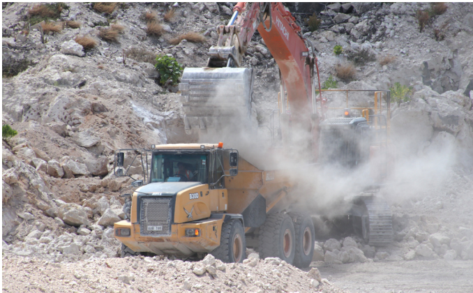
NRC machinery doing land clearing
