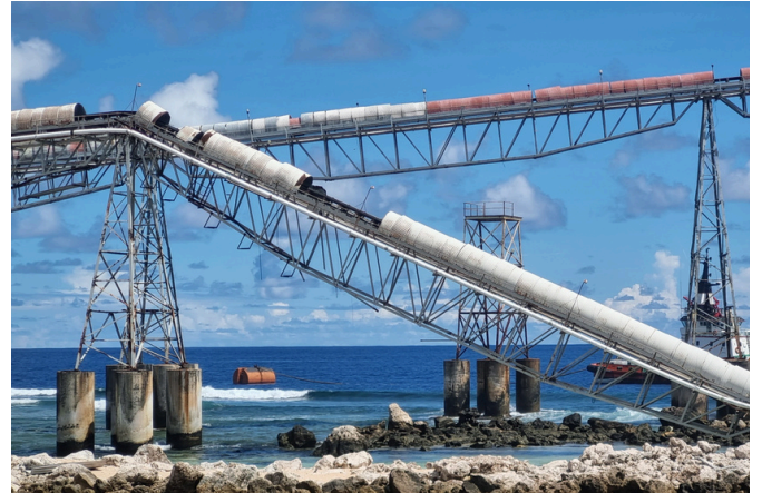
Ronphos focused on improving production, dust suppression works, and cantilever rebuild
