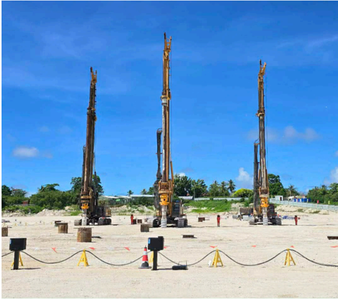
Specialised machinery carry out foundation work for stadium
