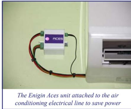
*The Enigin Aces unit attached to the air conditioning electrical line to save power*
